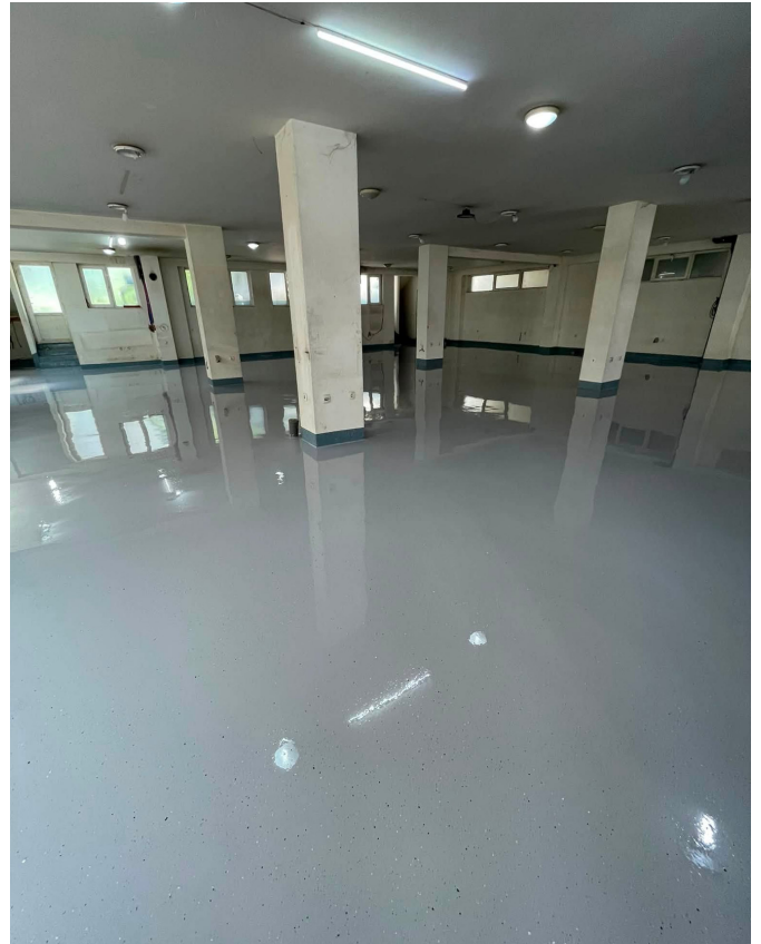
LARGE INTERIOR FLOOR AREA
